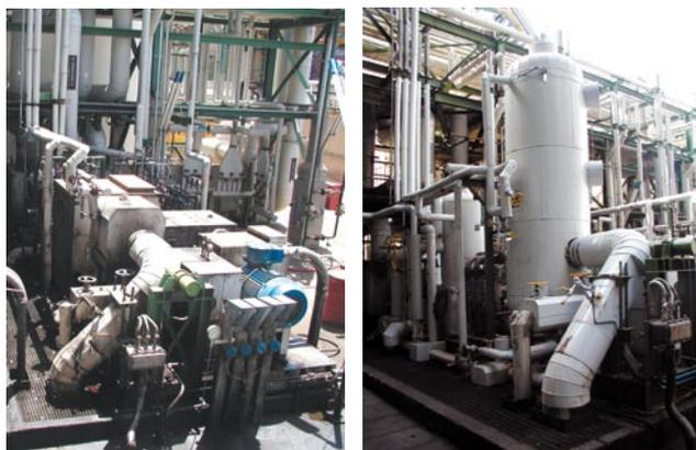
Figure 4. Picture of one pumping unit prior (left) and after (right) the plant modifications (in foreground: discharge side; in background: suction side). The suction dampener is approximately 2.5 m high; the discharge dampener is approximately 4 m high.
